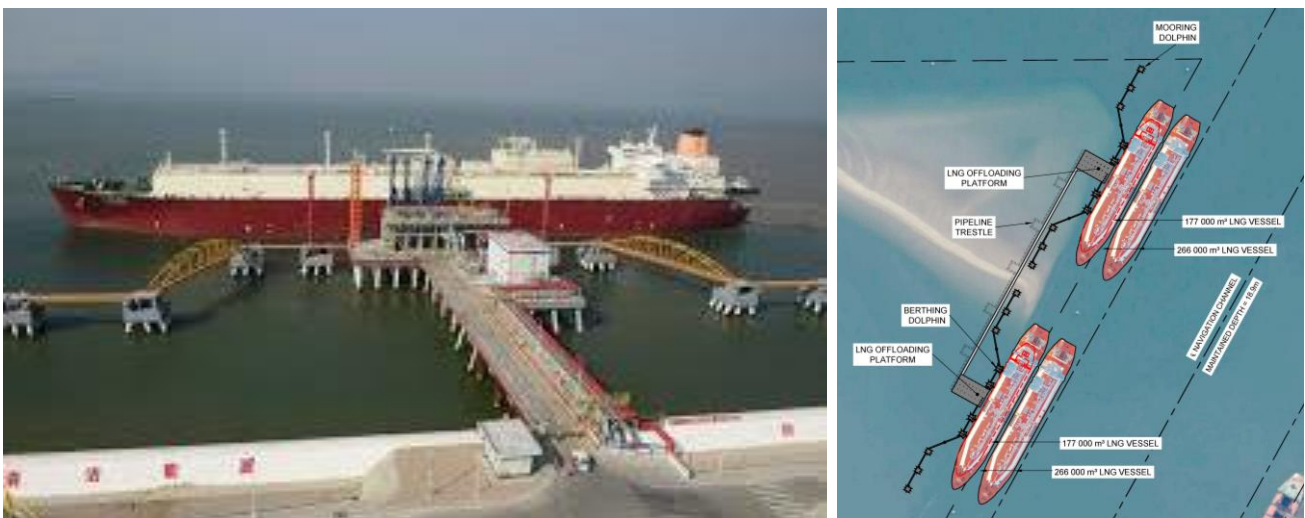
Figure 3: Left: Typical multiple piled concrete and steel quay; Right: Schematic design of the LNG Terminal capable of accommodating two LNG FSUs and/or vessels at the same time.
